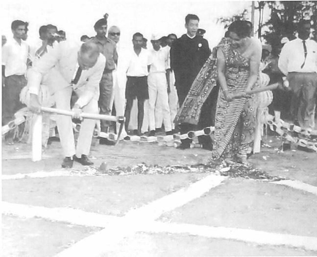
Prelude to the laying of the foundation stone for the Bandaranaike Memorial International Conference Hall, 1970.
